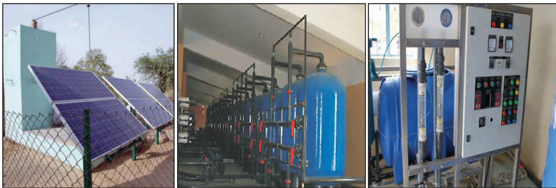
Figure 5.5: Solar-powered RO filtration plant
